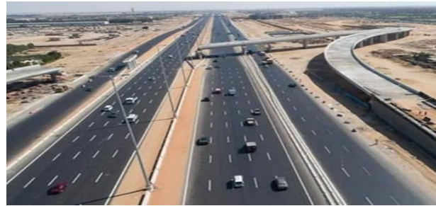
Figure 6. Photo of Egypt Highway Road
